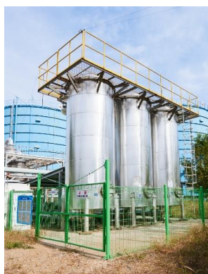
Tancheon water regeneration center (Seoul)
